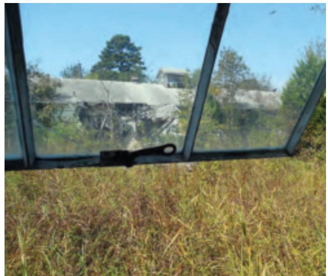
Part of Fort Chaffee Hospital complex still standing. Some of the buildings have burned. Photo by James Kirkendall
