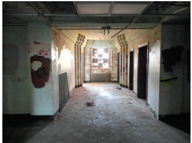
Art deco details in the 1909 Nyberg Building stand out even in its empty condition. Sanatorium photos by James Kirkendall
